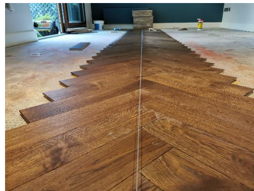
Figure 1. Engineered Herringbone Crown Row
